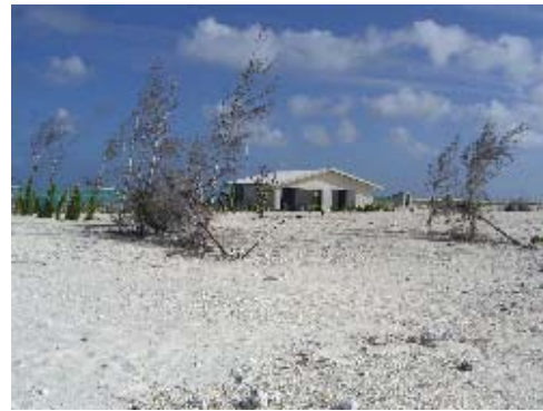
The 3B7C operating hut on Isle du Sud
